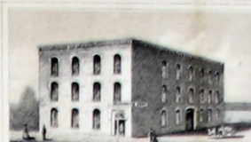
D. MIERSWA WAGON & PAINT SHOP.
