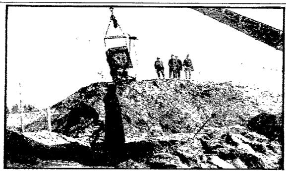
The dragline bucket has just dropped its load in place on a two mile dike, Job No. 17 in North Millston township, Jackson county, in Site 2 of the central Wisconsin game refuge. The job will require the moving of 45,000 cubic yards of dirt, making a dike averaging six feet high. It will have a four-foot top, and is built over galvanized wire netting to prevent muskrats from tunneling through. It will create one of the largest flowages in the refuge. About 90 flowages are planned.
